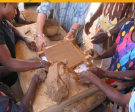
Logshegu village, North Ghana, our first experiment with floor and roof tiles
